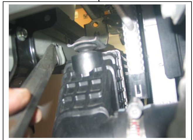
Figure 6: Chisel off temp sensor mount
